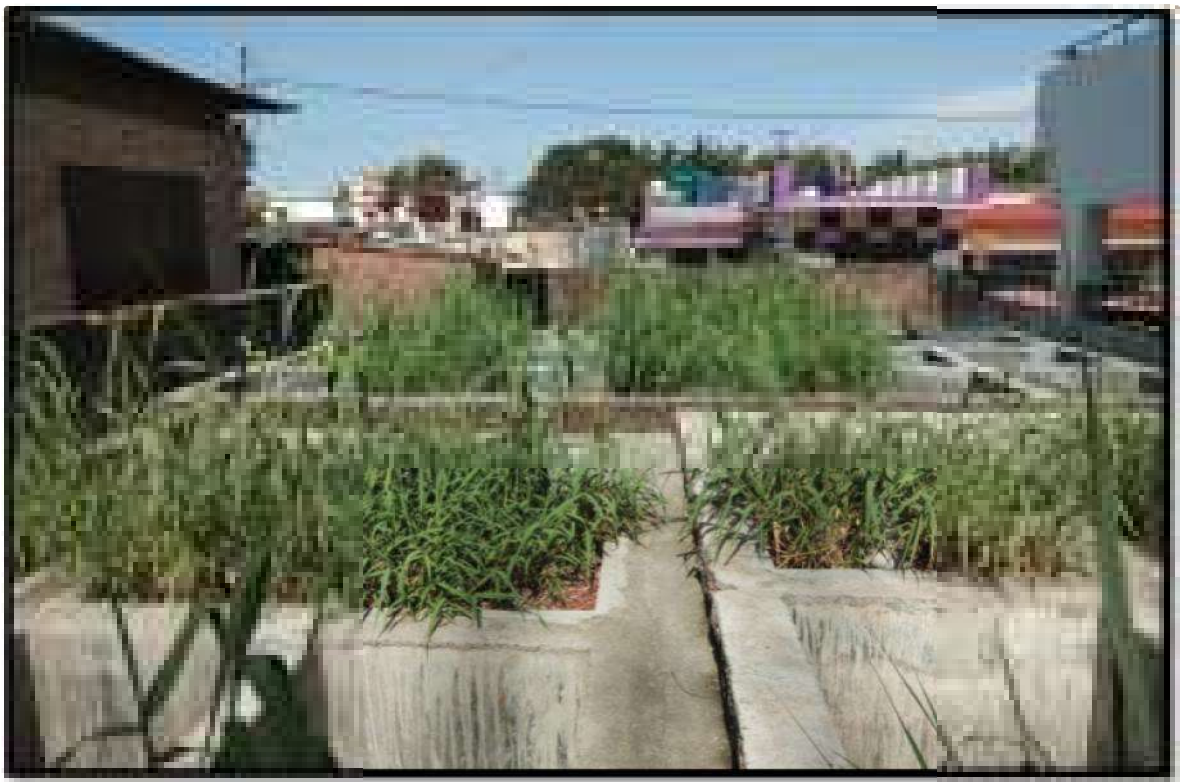
Dairy Waste Treatment Plant for treatment of Liquid Dairy Waste
